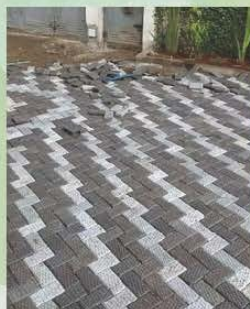
Recycled bricks produced by Gjenge Makers Ltd. being used to pave a driveway
