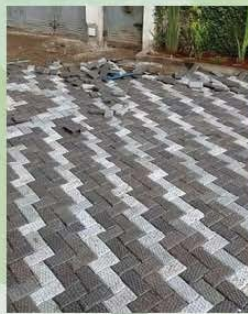
Recycled bricks produced by Genge Makers Ltd. being used to pave a driveway
